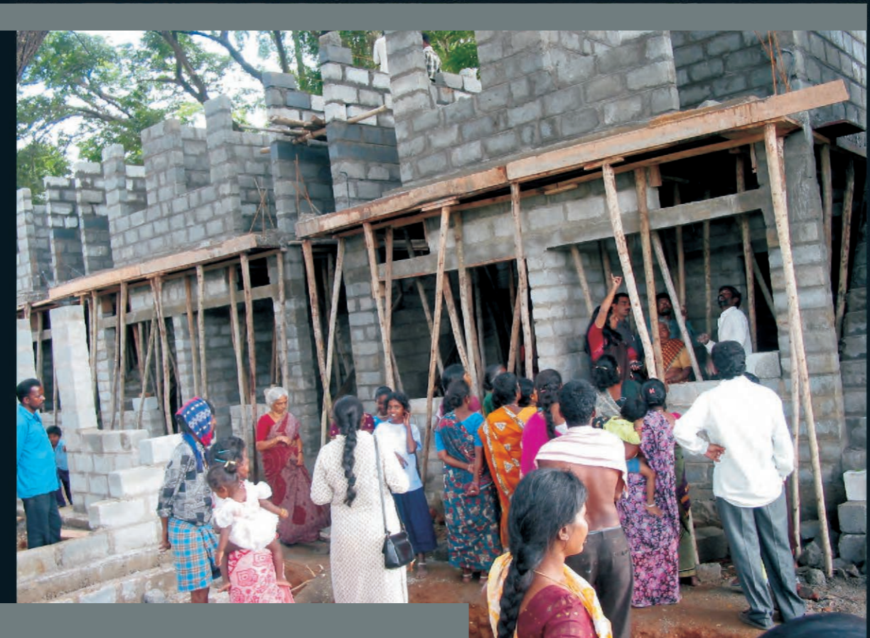
New homes being constructed in Sanyasikunte.
