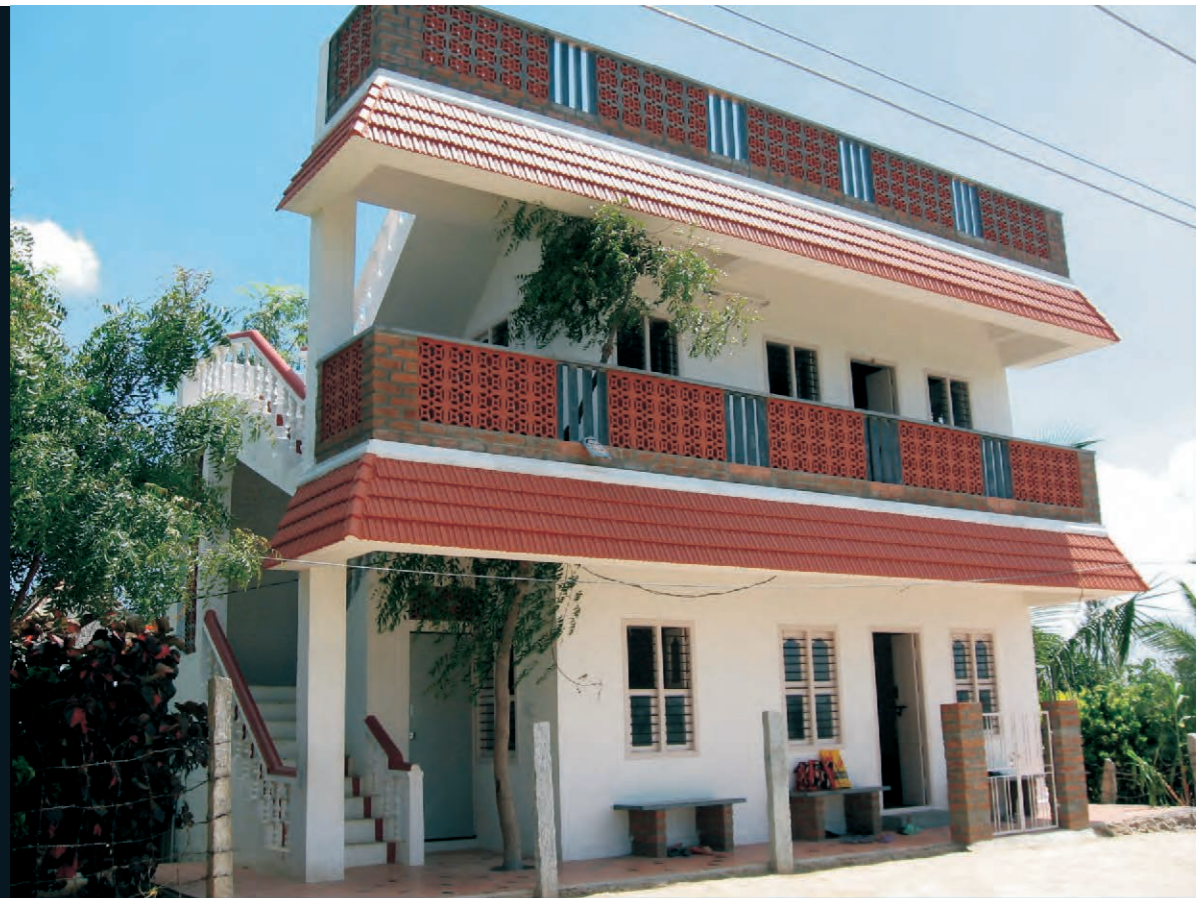
The SWECHA community centre, built by DRRT, for the development of the Sugali community.
