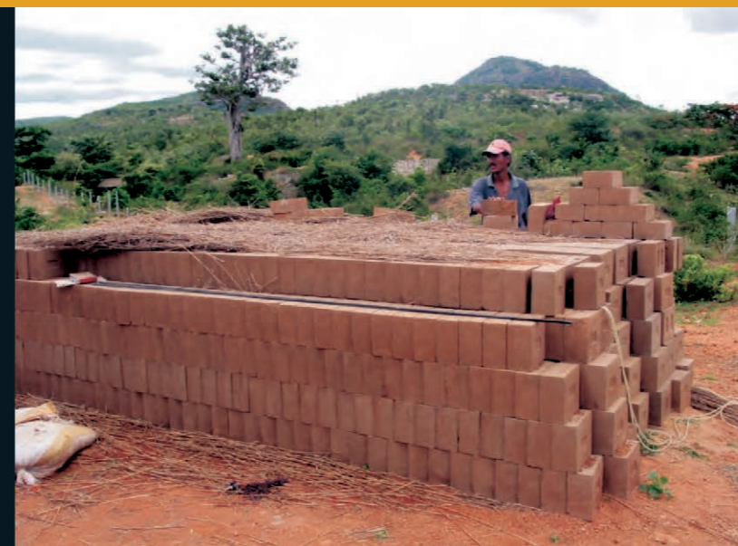
Soil stabilized bricks on site, promoting eco-conservation.
